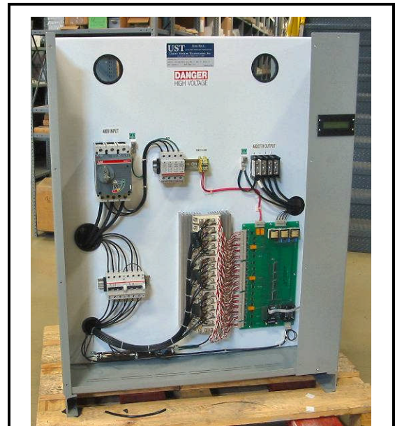
Controls and electronic switches in an electronic tap switching voltage regulator
